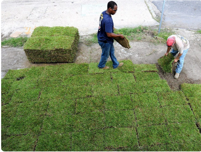
Reference: fresh-cut Bermuda rolls going down on a leveled base.
